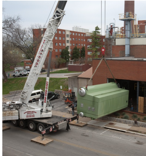
Installation of natural gas boiler, spring 2011.
