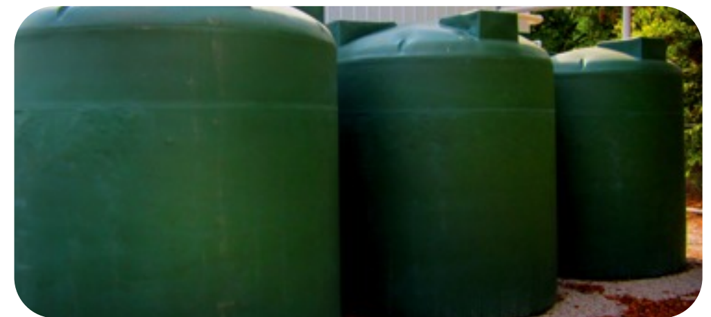
Six, twenty-six hundred gallon cisterns collect water from the Department of Facilities Management maintenance barn. This water is put onto a water truck to fill irrigation bags around campus trees.
