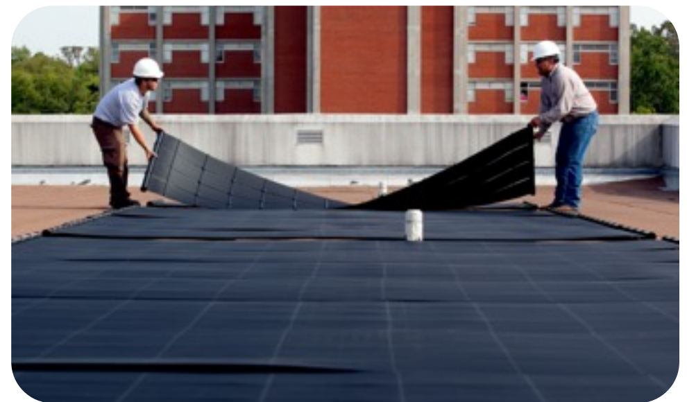
Installation of the solar thermal array. Photo by Clinton Lewis.
