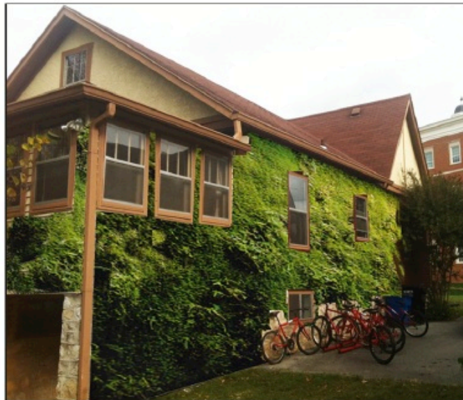
South-east facing side of house with Green Screen. The trellis system supports the plants so that the root won't damage the structure. It really makes it a 'Green House'
