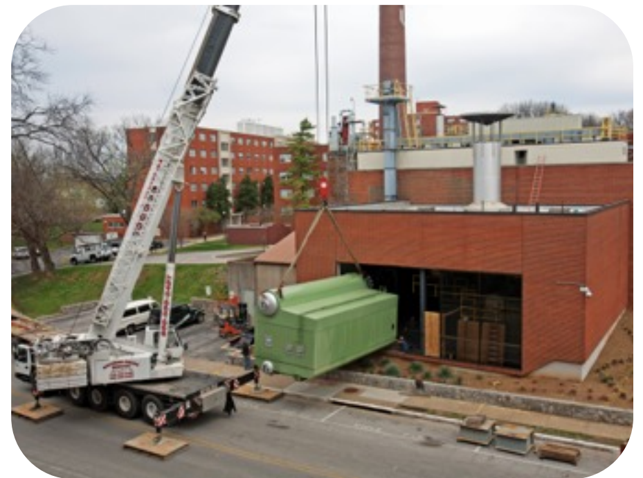
The first of the natural gas boilers, being installed in 2010. Photo by Clinton Lewis. Click to read more about WKU installing large natural gas boiler at Central Heat Plant .
