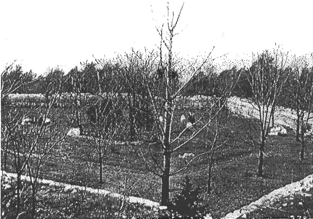
Figure 7. A 1907 view of the interior stone walls of the fort; walls appear to be intact in this photo taken from Potter Hall, facing north, northwest; note west wall in rear center and left of photo.
