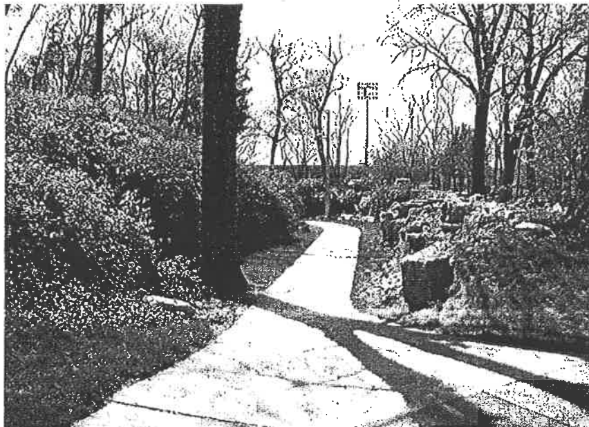
Figure 11. View of trench and sidewalk along the outside of the "west" wall, facing southwest. Blasting drill holes were visible in the bedrock exposures to right.
