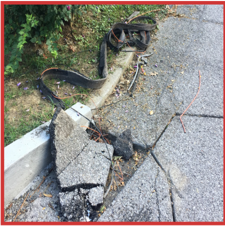
Fiber Restoration Project Corner of Dundee and Fleming Rd.
