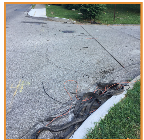
Fiber Restoration Project Corner of Dundee and Fleming Rd.
