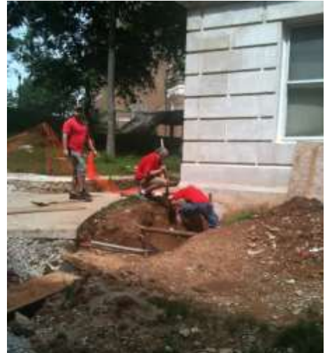
Removed old water line and hydrants at Gordon
