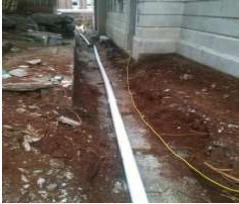
Gordon Wilson –Repaired domestic water line and worked with contractor with removing old piping.
