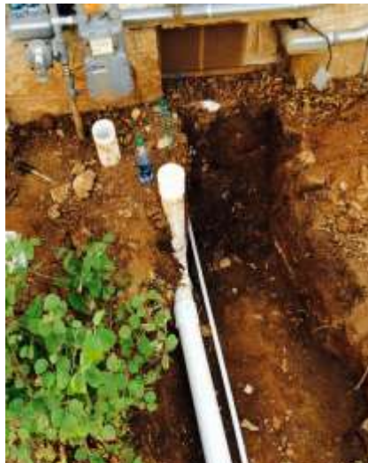
Replaced sewer and water line at 1702 Normal Dr.
