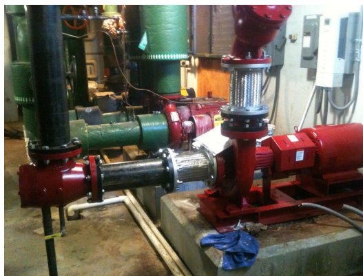
Installation of new chill water pump.
