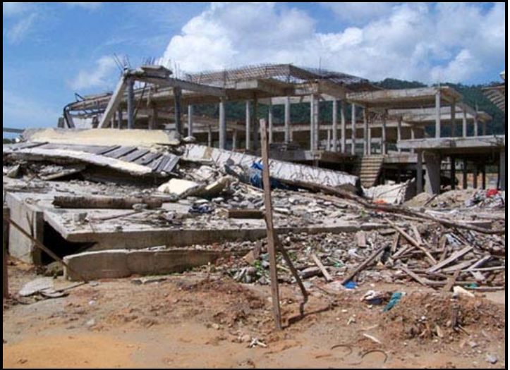
Wreckage from the Tsunami
