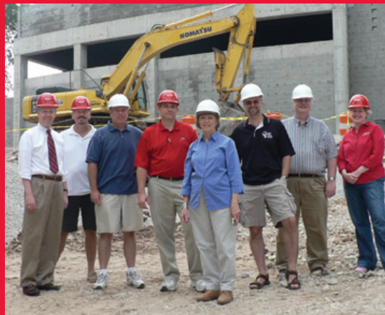
New music hall construction site, l to r: David Lee, Marshall Scott, Gary Schallert, Jeff Bright, Mitzi Groom, Paul Hondorp, Joe Stites, Mina Doerner
