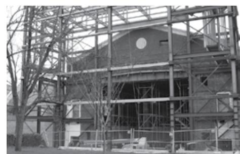
A new back wall that is thirty feet higher than the original has been added, along with new 2008-09 construction on the side to accommodate dressing rooms, a multipurpose staging room and a green room.
