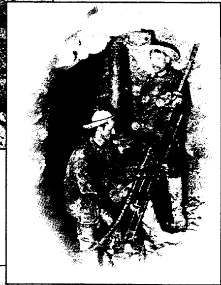
Miners drifting (that is, following the vein) 2,100 feet underground with an air-driven machine drill, Nevada County, Empire Mine, 1900. G.W. Starr Collection. DMG photo A7151.
