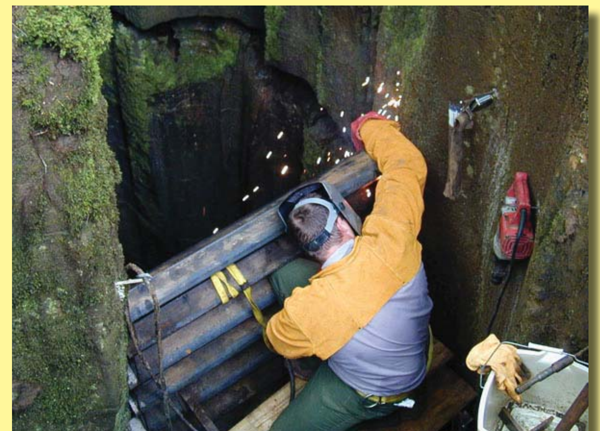
A volunteer works on a cave gating project.
