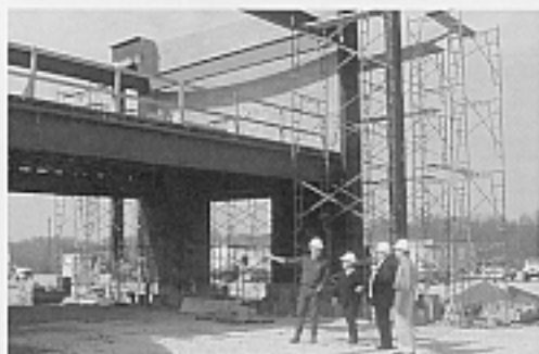
The new Glasgow Library under construction
