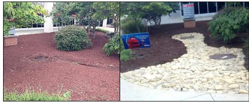
communication, coordination and cooperation between grounds, maintenance, building services and PDC. By recording the data, monitoring our corrective efforts and being apprised to approaching weather conditions. Many of the existing ground level storm drains have been subject to contamination such as leaves, mulch trash and other materials. One way to help minimize this is to enhance the run-off channels and create deliberate swales for the storm water to flow through
