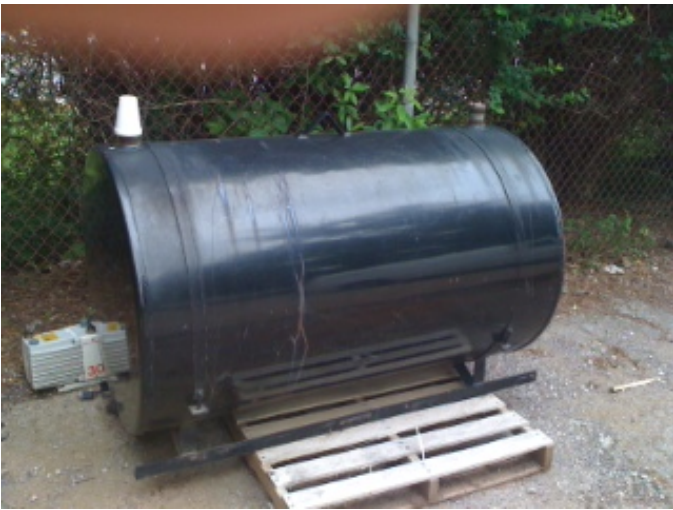
Fuel tank (had diesel in it)
