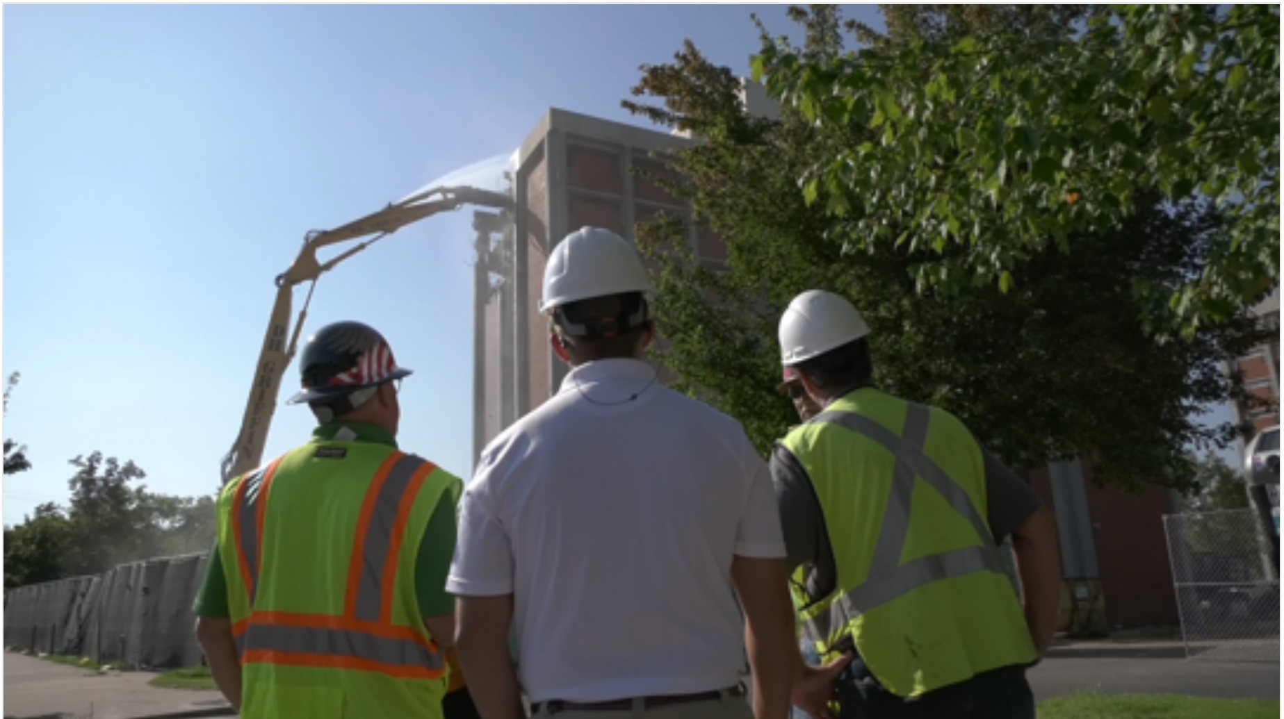
VIDEO: Demolition begins for First Year Village at WKU
